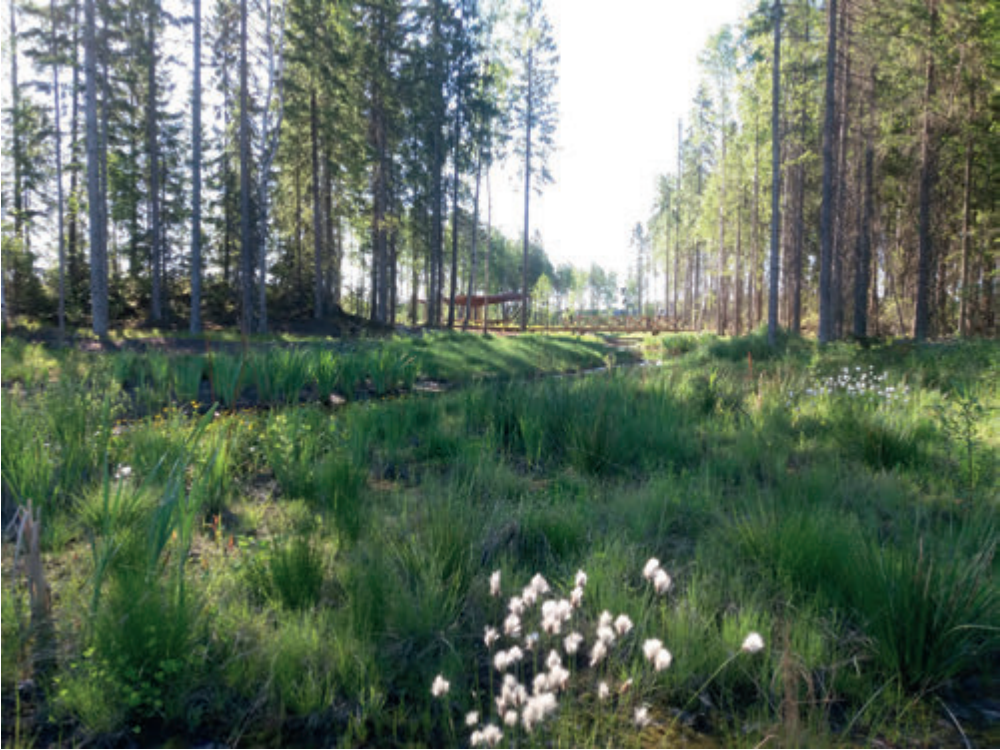
Figure 1. A constructed wetland in Vuores, Tampere, filters stormwater runoff to remove pollutants before discharge to the area's oligotrophic surface waters. Image © Maarit Särkilahti.
