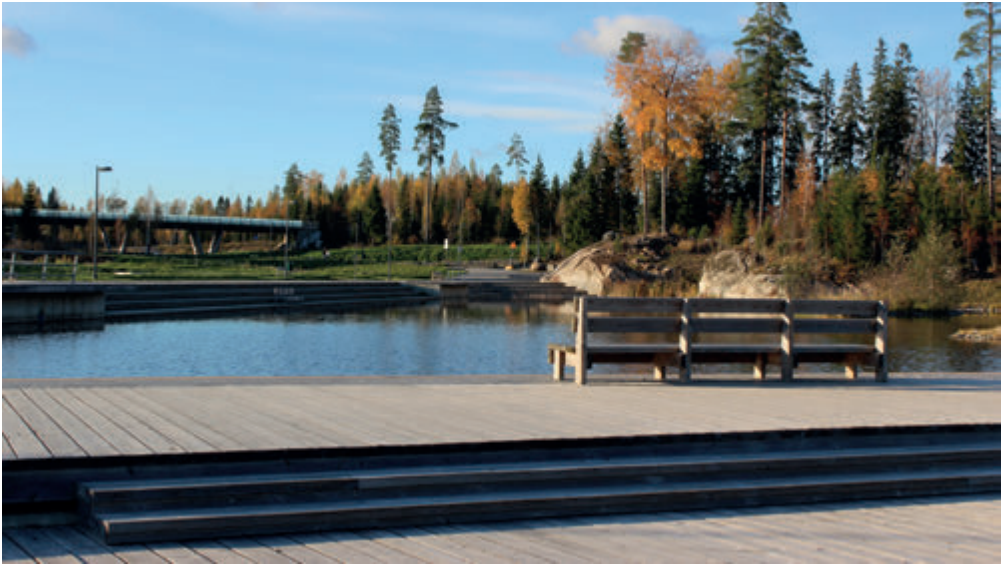
Figure 3. The heart of Vuores' nature-based stormwater management system is Central Park, where retention ponds (above), swales, and wetlands retain and purify waters before discharge to Lake Koipjärvi. Image © City of Tampere / Vuores
